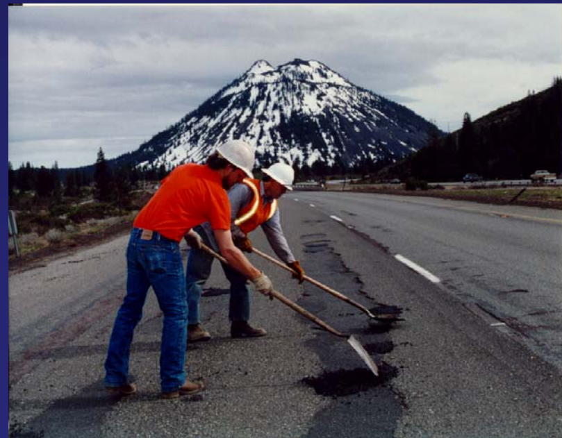
Caltrans Road Maintenance Siskiyou County
